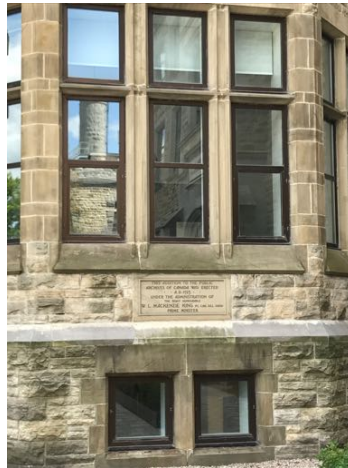
Figure 8.4: Global Centre for Pluralism additional wing Credit: Sahir Dewji
