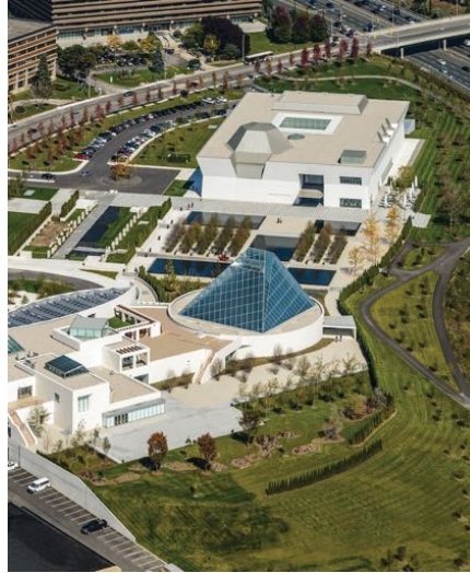
Figure 9.4: Aerial view capturing the landscaping, buildings and pools Credit: © The Ismaili Canada
