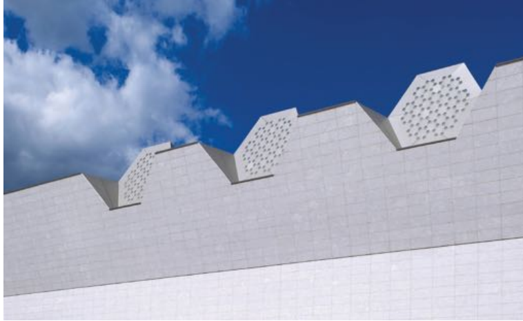
Figure 9.3: Exterior view of the skylights at the AKM Credit: © The Ismaili Canada
