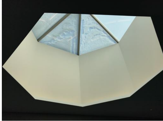
Figure 9.2: Skylight above stairs Credit: Sahir Dewji
