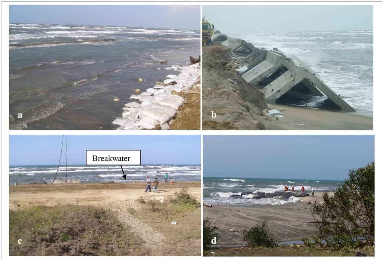
Figure 5. Shore protection measures installed at the 20<sup>th</sup> km. a,b,c. Breakwater made with panels of reinforced concrete (Photos taken in April, 2011 by author). d Sandbags installed to trap sediment (Photo taken from the road toward the northeast on May 28<sup>th</sup>, 2014 by Cristóbal Pizarro).
