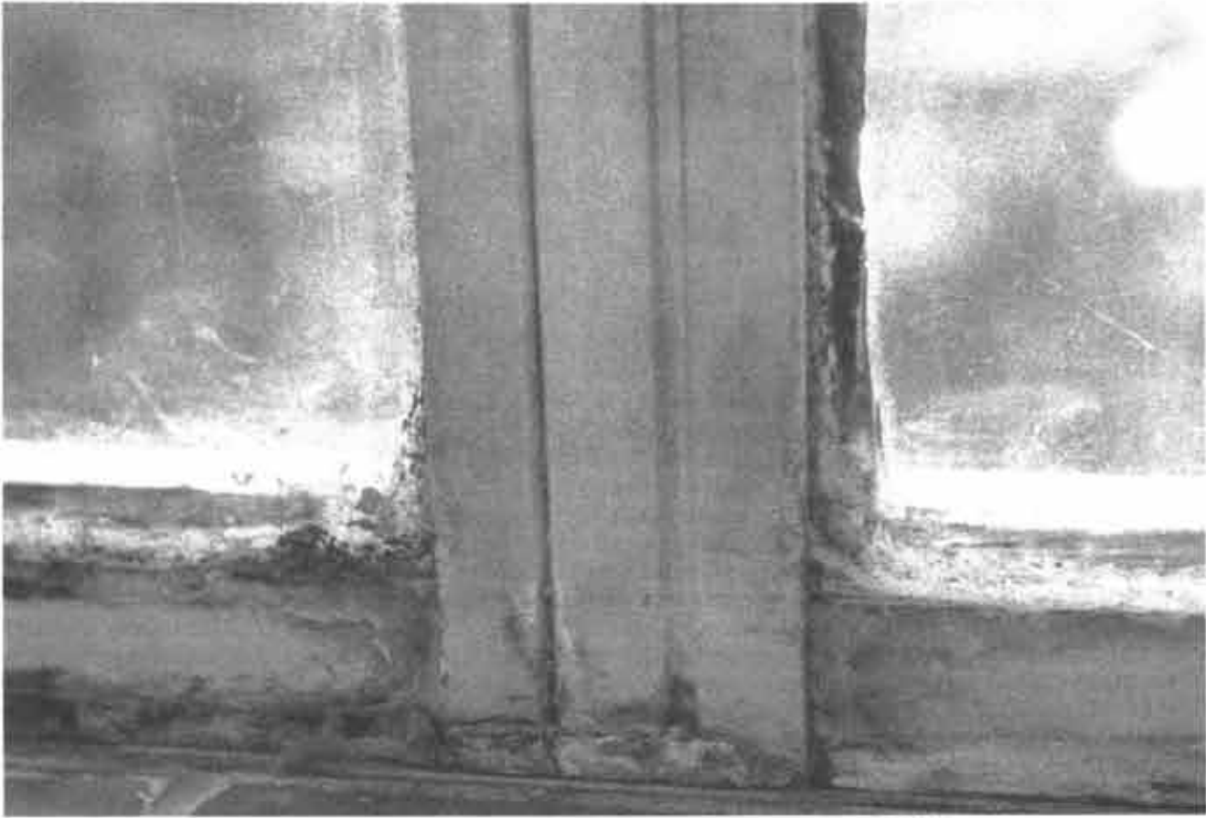
A window frame in the Arts building shows signs of corrosion. These particular windows are among those classified as "end of life" and recommended for replacement by the energy management plan.
