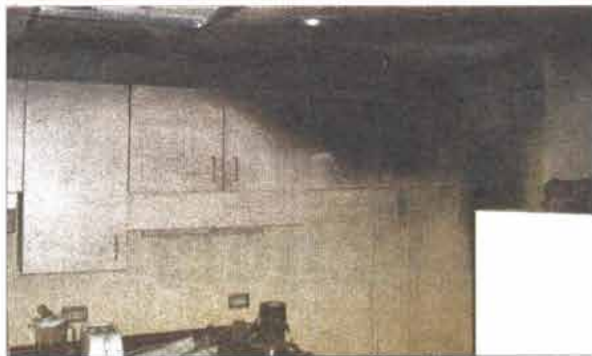
SMOKED OUT - Top: The light bulb from a residence fridge ignited a sofa cushion. Bottom: Smoke damage from the fridge fire.
