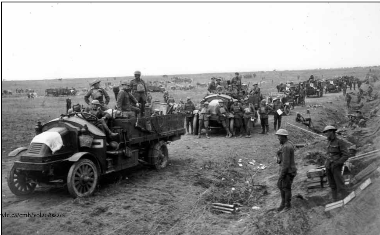
A column of vehicles belonging to the Canadian Motor Machine Gun Brigade waiting alongside the Arras-Cambrai road, September 1918.
