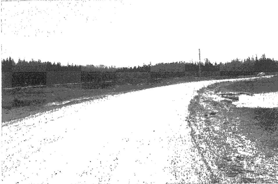
Figure 5.7 Supplying Lake water to a Confined Wetland Zone with a piping system underneath Shoreline Ave. (Tupman, 04-22-2002)
