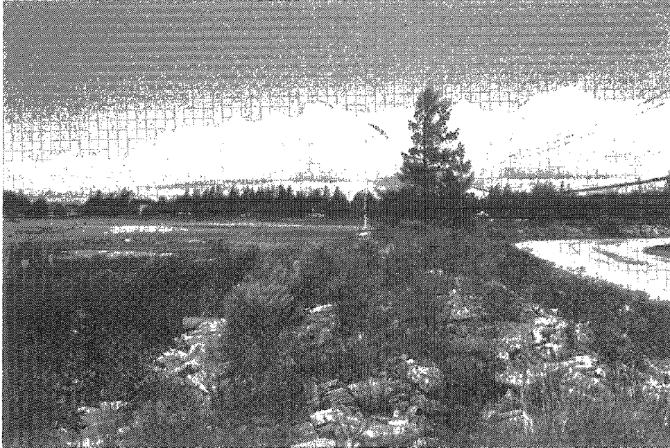
Figure 5.6 Shoreline Hardening in Oliphant. Shoreline Ave to the right. Shoreline hardening was established in late 1980s after record high water levels. Water level is clearly low, as it is not visible. (Tupman, 08-25-2002)
