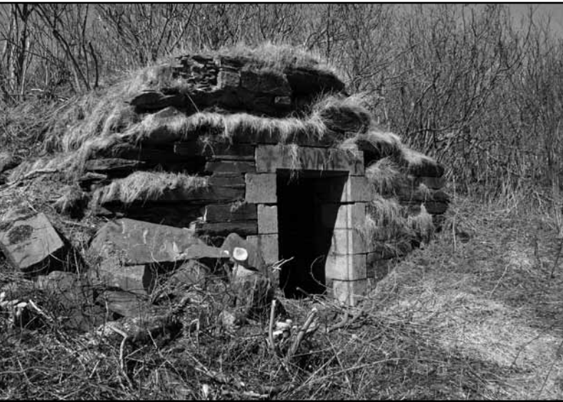
Above: The entrance to the southern expense magazine. Note the heavy earth cover over top of the magazine.
