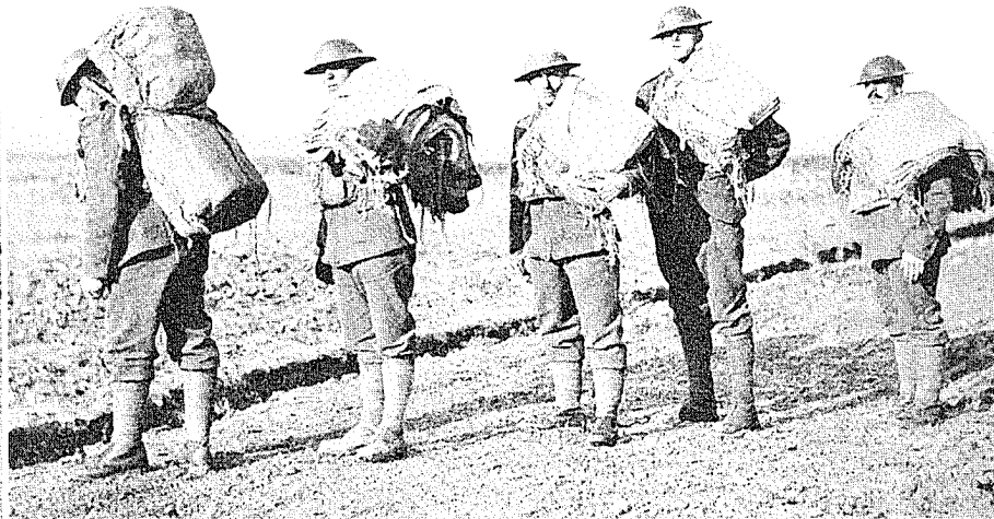
Nature of Load: 1 bale of sandbags Weight of Load: 115 lbs. (dry) Usual Carrying Party: 4 men Percentage saved in manpower by use of tumpline: 75 percent
