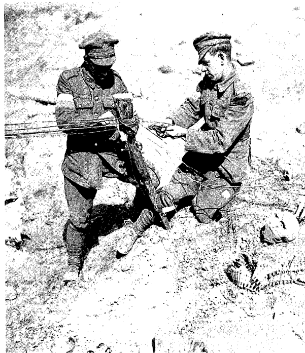
To keep wires off the ground Canadian Signallers use a German rifle as a telephone pole. September 1918. NAC PA 3100
