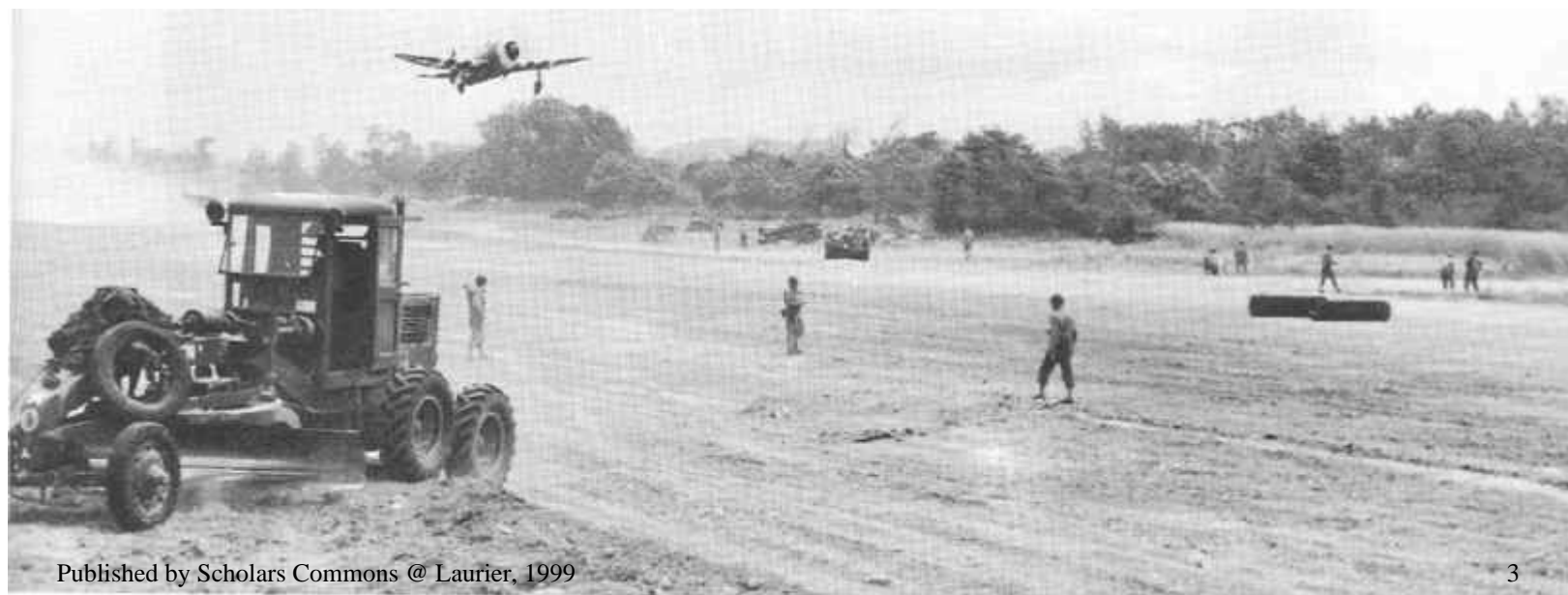
A P-47 Thunderbolt takes off from a frontline landing strip after being refuelled and rearmed by mechanics of the 9th Air Force Service Command. The strip is still in process of construction and work goes on despite aircraft landing and taking off. (USAF Photo PRO HQ 44-1533)
