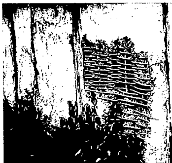
Fig. 2: Wattle and daub construction, Jamestown
