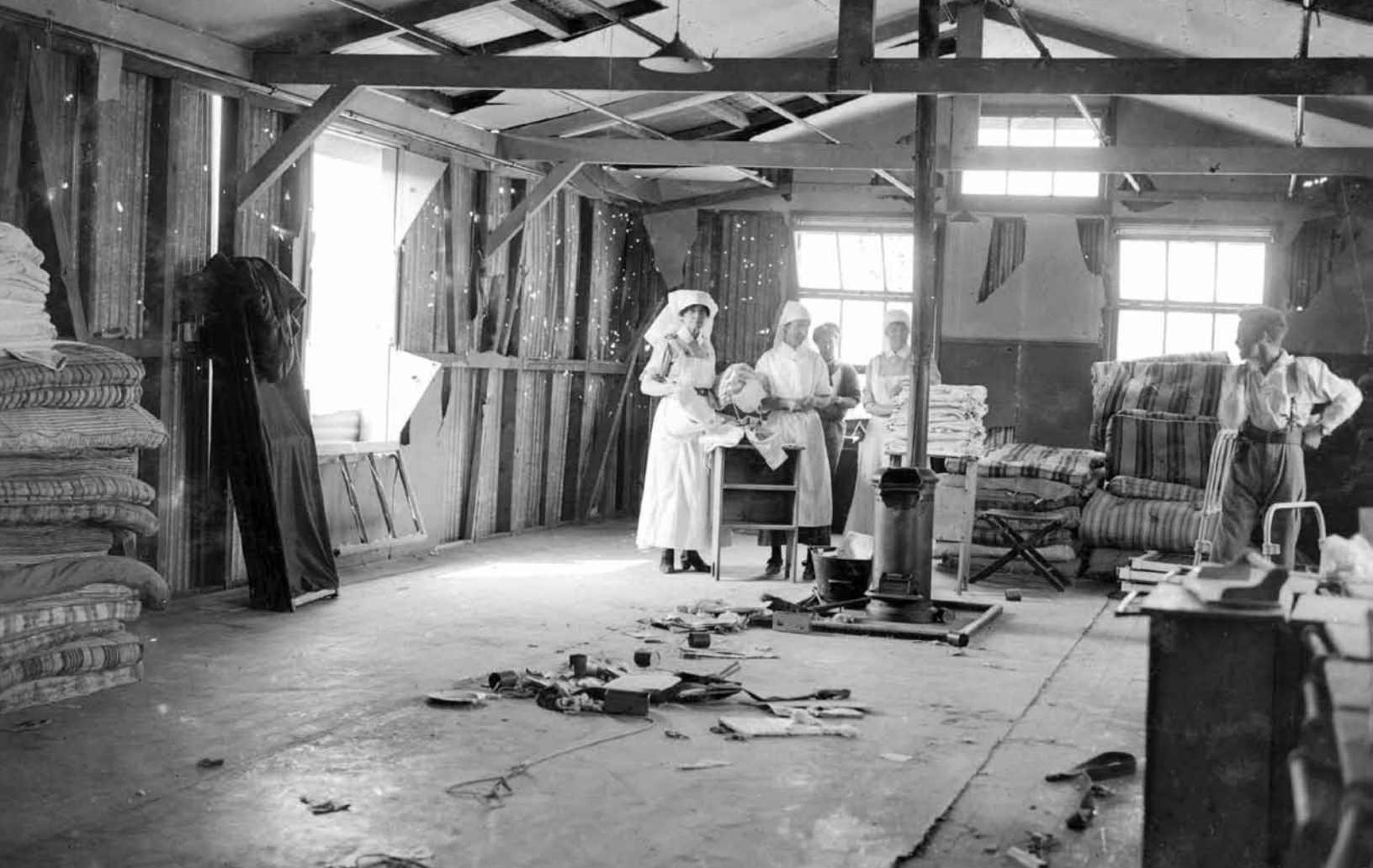
Canadian nursing sisters cleaning up ward of hospital after an unidentified bombing raid. Note the multiple perforations in the tin wall caused by the bomb blast.
